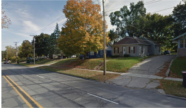
EXISTING SITE near Sta. 42+00 908 & 904 West 1st Street
